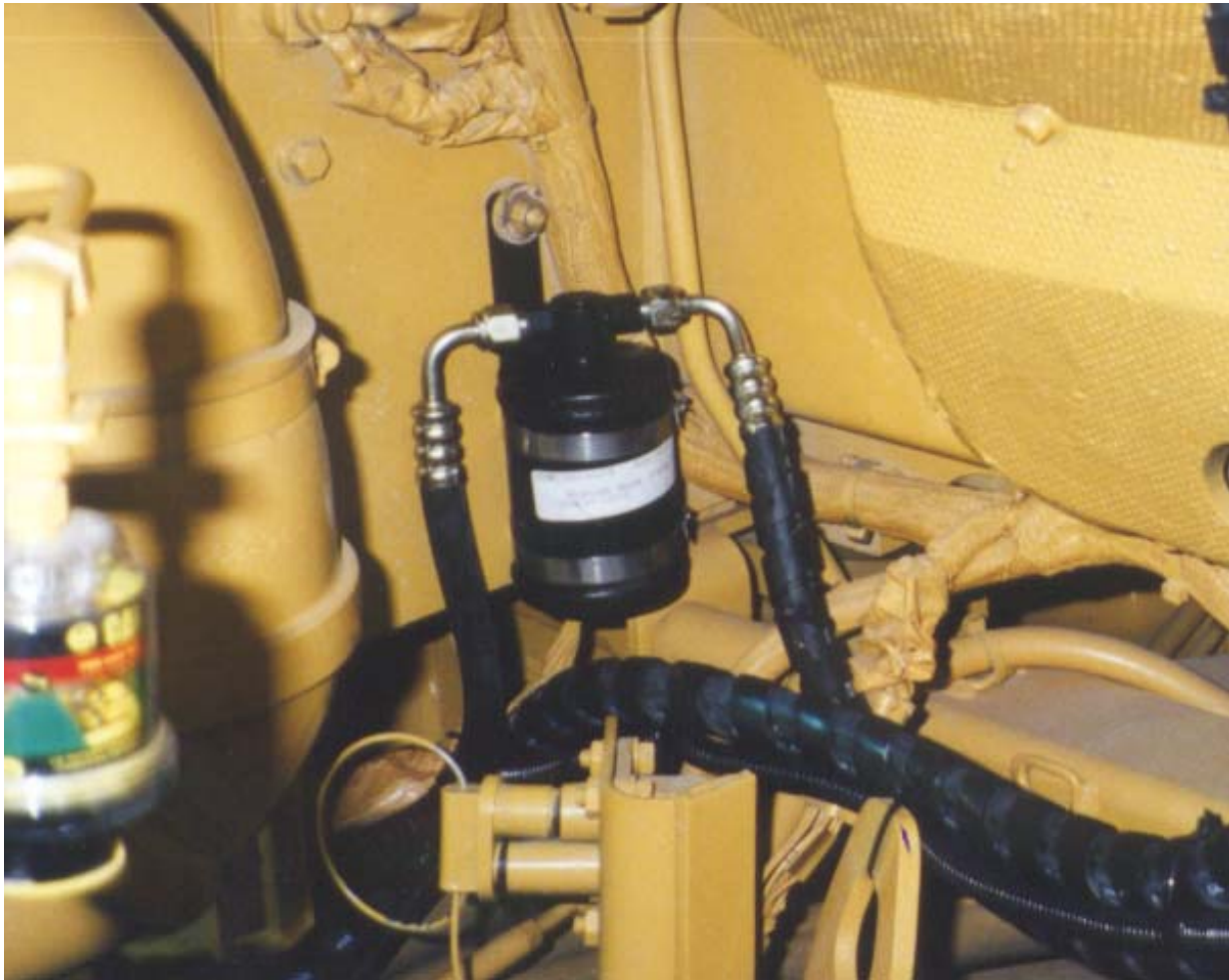
Drier and hoses in place.
